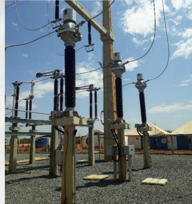
Oil-Insulated Current Transformers 72.5 kV to 800 kV, up to 5000A
